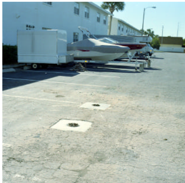
Completed Monitor Wells, February 1996
