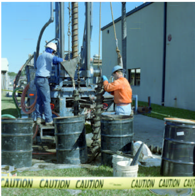
Monitor Well Installation, February 1996
