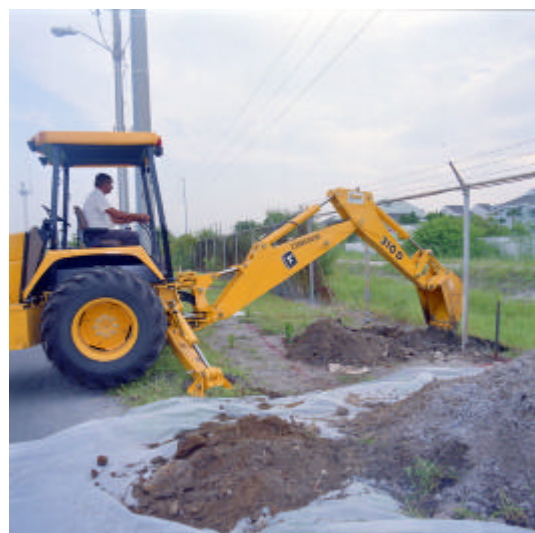
Contaminated Soil Removal, August 1992
