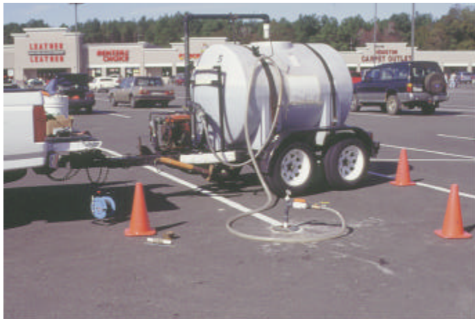
Bioremediation Nutrient Injection System, Houston TX
